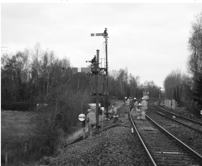
**Construction company Eric Wright Civil Engineering installed new semaphore signals at Howe and Co's Sidings during April; they are in the foreground and replace the tall 'bracket' signal behind. Also visible is Howe and Co's sidings signalbox which was installed by the Midland Railway in 1912 and which is expected to survive for a time after the closure of the rest of the S&C's signalboxes.**
